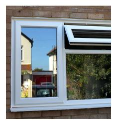
IMPORTANT NOTE: If non-locking handles are required, and any windows/tilt & turns are adjacent to a door, one pane of glass must be laminated to BS EN 356:2000 Class P1A
