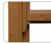
Run through sash horns
