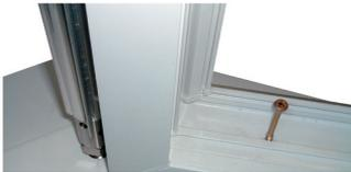
**8)** Fix down through the frame into the cill, with the frame tight against the cill upstand. Follow your normal fixing guidelines in terms of screw types and fixing centres.
