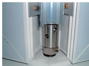
**11)** Cut the internal trim to size and clip into position. This will centralise the assembly and assist before you screw fix the baypole to the frames. The trim should locate neatly on top of the window board or cill upstand. Before clipping into position, you have an option to run a bead of sealant into the 'cups' along the edge of the extrusion for additional weatherability.
