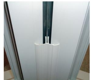
**13)** When all fixings are in position, cut the outer trim to size and clip it into position. You can also run a bead of sealant along the edges if you wish - prior to fitting. Protective tape is supplied and this should be removed within a day or two of the installation. Finish the installation as normal.
